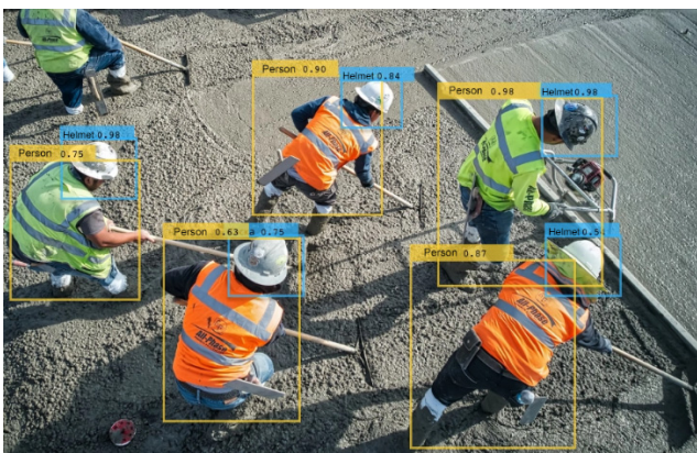
Fig. 1 – Employee safety control
